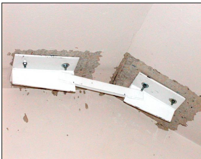
▲ Zhotovenie kotvenia K2 Preparation of K2 anchorage
