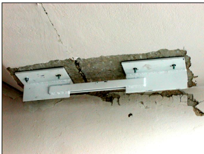
▲ Zhotovenie kotvenia K1 Preparation of K1 anchorage
